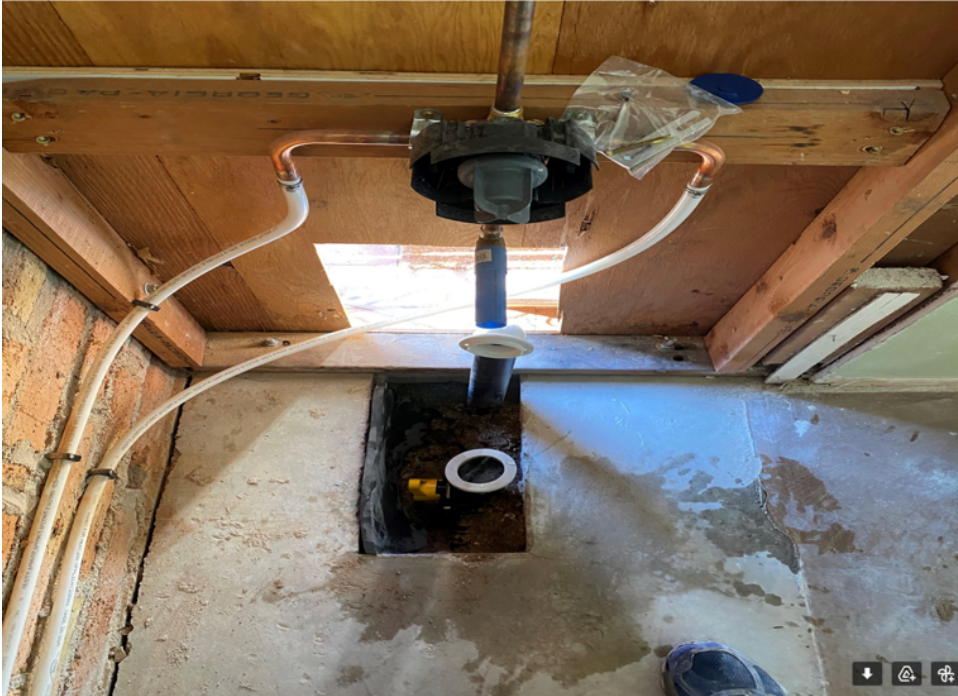
Valve installed under the bathtub, before tub installed
