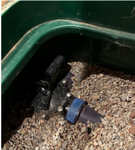
Close up of RB's three-way diverter valve allowing her to direct greywater to the landscape or the sewer.
