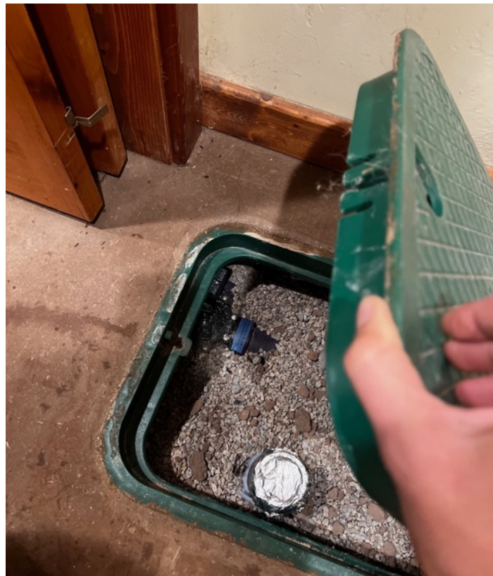
RB's 3-way diverter valve accessed via a valve box in floor of home
