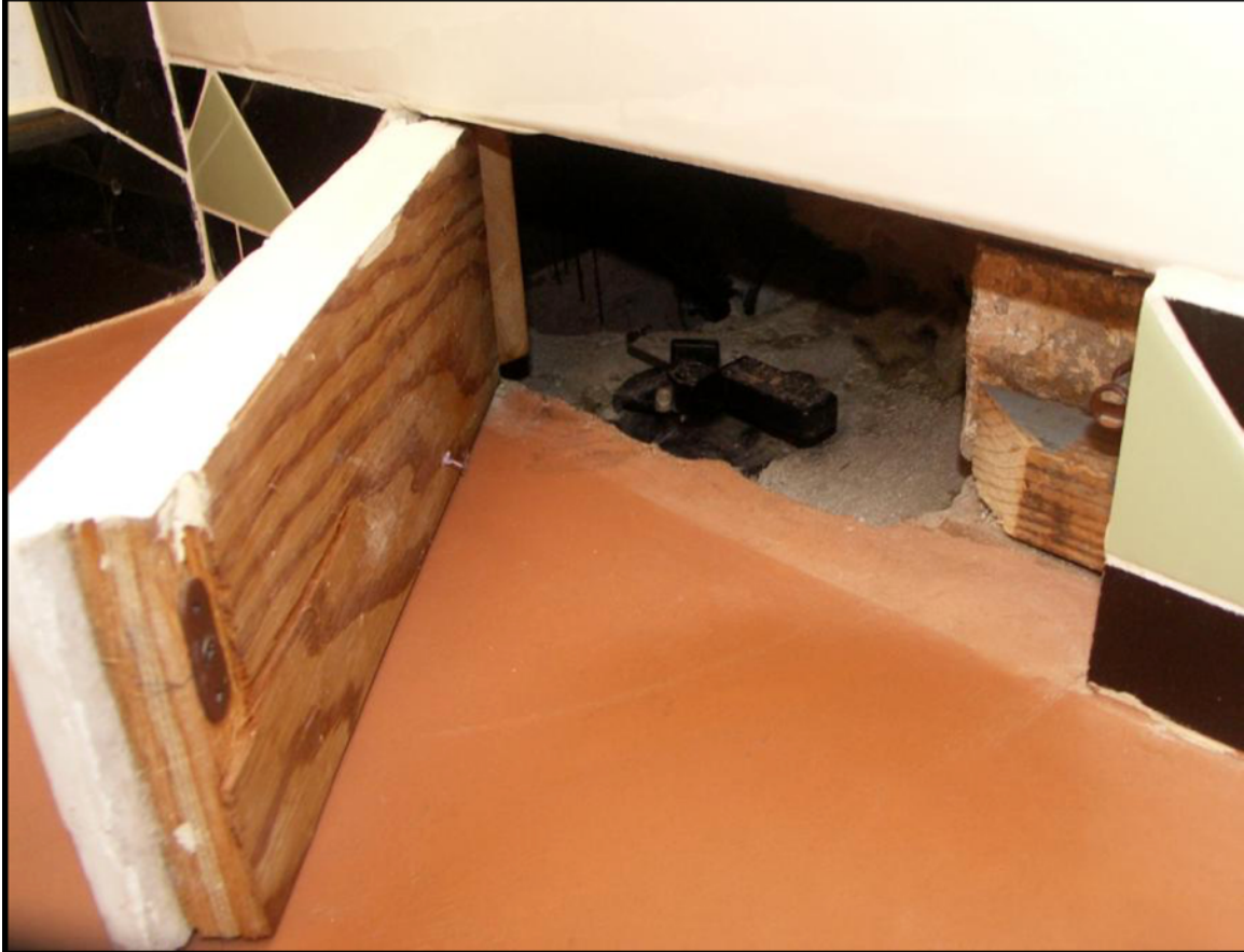
Close up of the three-way valve accessed via trap door under tub.
