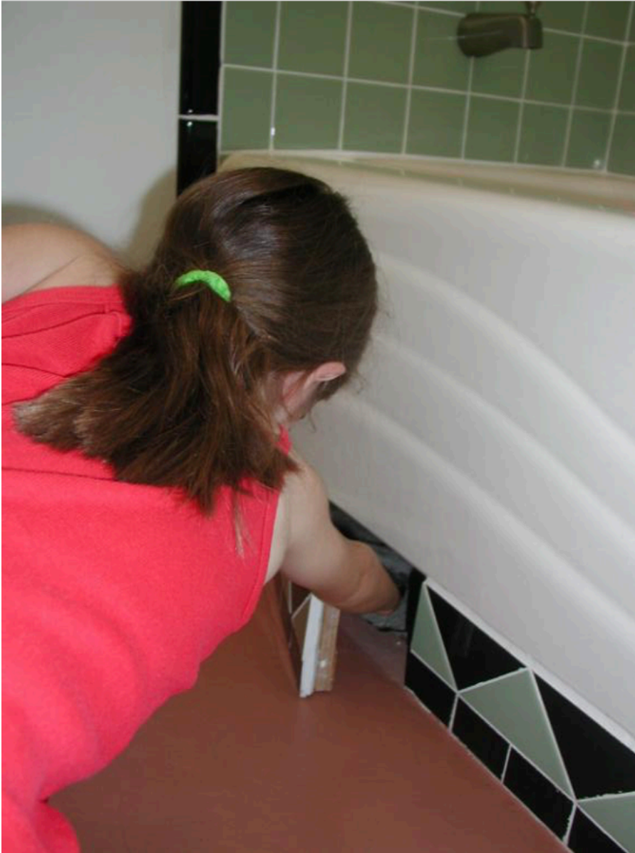
Accessing bathtub three-way diverter valve via trap door under tub at SN residence.
