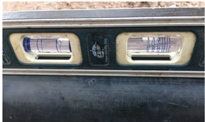
Fig. A1.14B. Close up of level reading drop/slope of 1/4-inch drop per linear foot. Note how the right edge of the bubble on right vial touches and reads 1/4-inch slope.
