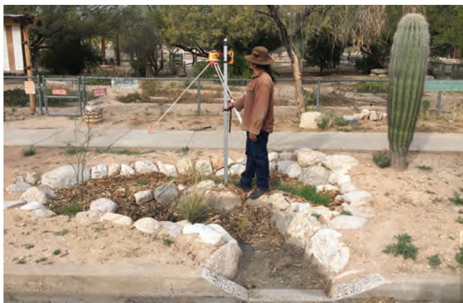
Fig. A1.11C. Omar is taking an elevation measurement on the planting terrace of the rain garden's infiltration basin. Ideally, the top of the terrace is built no higher than the elevation of the curb cut inlet so storm-captured runoff will rise to the top of the terrace, saturating it and the plants' root zone.
