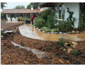
A swale infiltrates rooftop rainwater from the downspout at right and the walkway. Rainwater infiltration should be sited at least 8 ft from the foundation.
