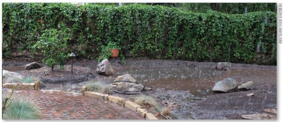
The ideal shape for infiltration: shallow, flat-bottomed basins below the grade of the surroundings, with low berms surrounding each basin, like dry rice paddies that fill only in storms. The basin above is in welldraining soil above a groundwater recharge zone. Minutes after this downpour stopped, the standing water had infiltrated.
