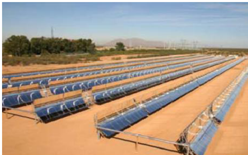
Figure 2. APS Saguaro Solar Facility, Red Rock, Arizona. Solar thermal plants like this one use water for cooling and mirror washing.
